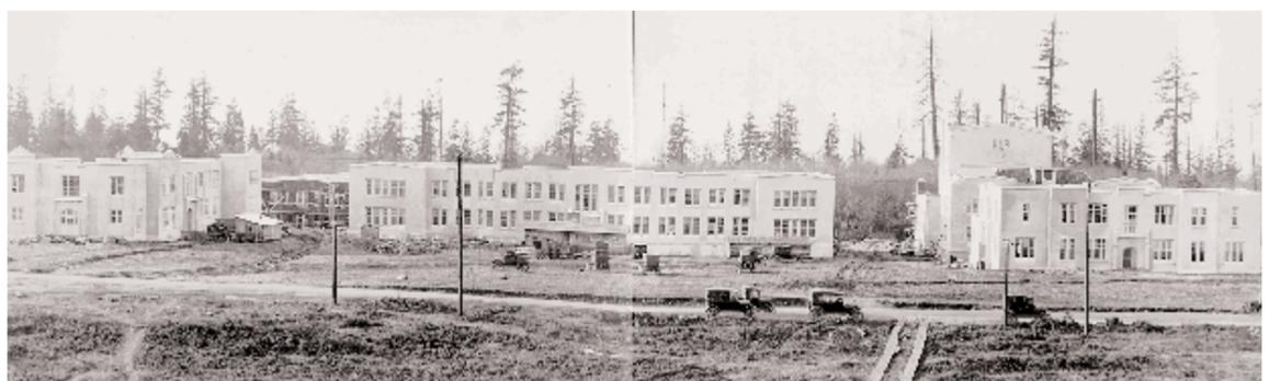
Semi-permanent buildings (left to right, Agriculture, Arts, Auditorium, Administration) under construction. Dogged by financial constraints in 1925, nine buildings, all of wood-frame and stucco construction were classed as "semi-permanent" and designed to last 25 to 40 years "if necessary." (As of 1996, most were still in use.) □
