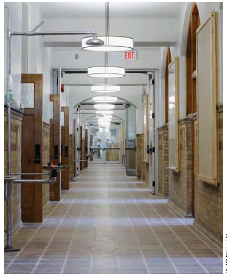
Chemistry Building renovation retains history.
